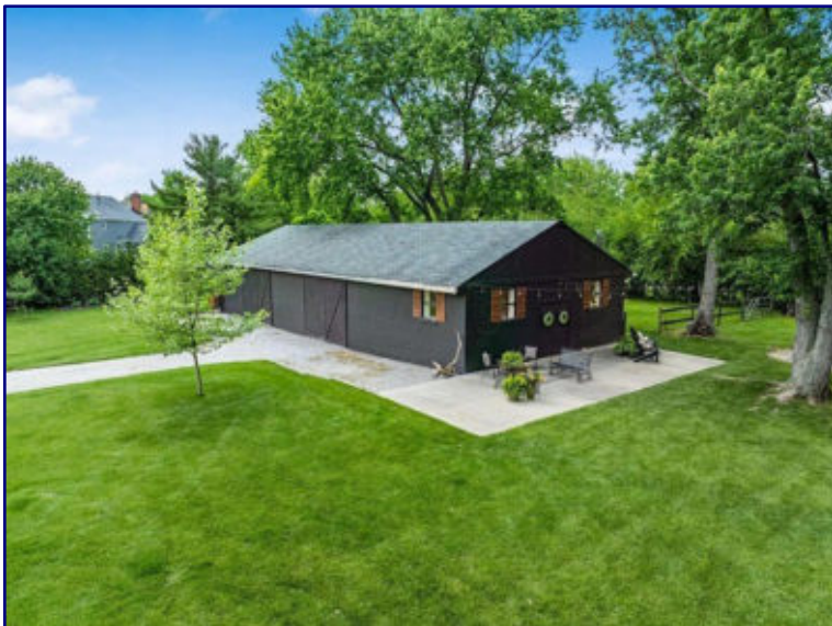
This is what the new building that Ztrack is currently moving into looks like. Photo: Ztrack
