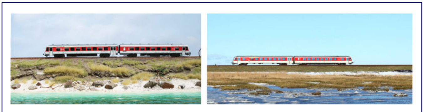
The Hindenburgdamm leading to the island of Sylt with a Class 628 multiple unit in the model (left) and as a prototype (right) exemplifies layout proposal 2 on page 23.
