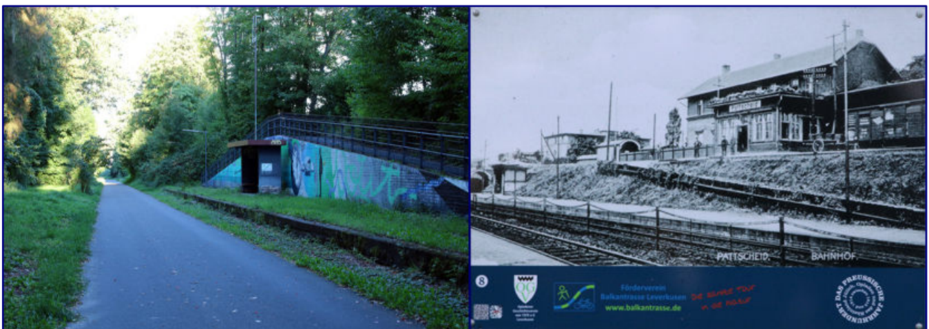
Two views of the exemplary restored Pattscheid station building (photo above). The view of the former track and platform at Pattscheid station in the direction of Opladen can now be seen from a cycle path. A plaque commemorates the original condition (Photo below).
